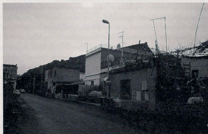
4. Urban expansion in the popular borgata on the via Casilina in Rome; after twenty years spontaneous buildings have assumed a consolidated image. Photo Simona Salvo.
