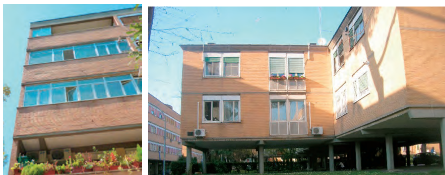
Figure 4 – Closed off balconies with different types of windows (left) and the addition of air conditioners
