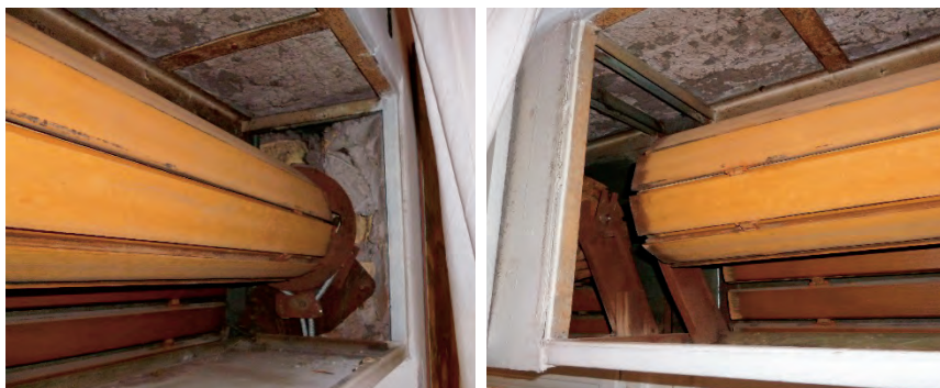
Figure 8 – Detail of the box and roll-down blinds
